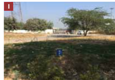
Entry to DTC Millenium Depot at Junction
