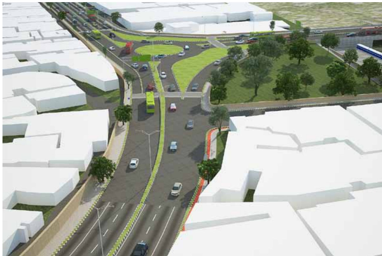
View of Kamal T-point from Sarai Rohilla Railway towards Anand Parbat View shows Table Top crossing at the junction and segregated lane for straight moving traffic towards Zakhira.
