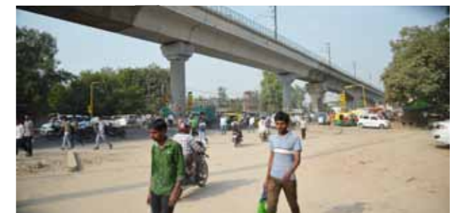
Encroachment of pedestrian phase in signal cycle by the informal streams of vehicular traffic from the depot results in unsafe and haphazard pedestrian crossing
