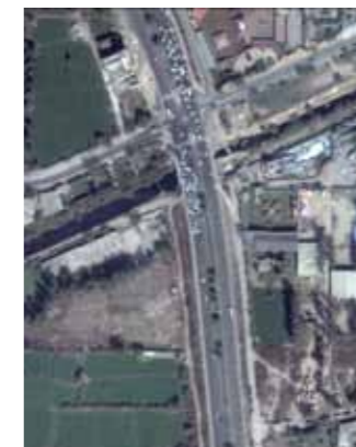
2012 - Slip road metalled on the other end of junction
