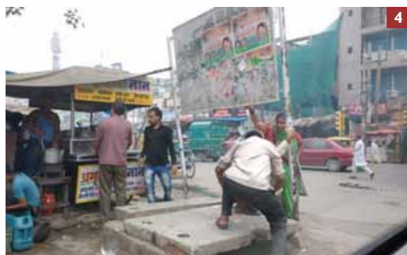
Concrete structure on the corner leading to insufficient turning radius for vehicles
