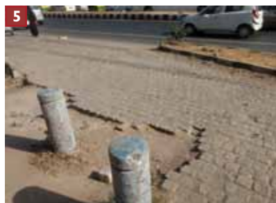
Broken and un-maintained footpaths
