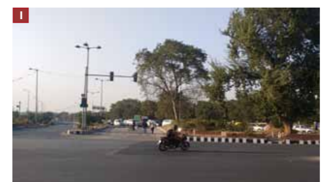
At grade arm at Junction leading to Dwarka : access to junction from the arm is blocked to reduce the signal cycle time as well as prevent heavy vehicles from entering the T3 underpass further ahead of the junction
