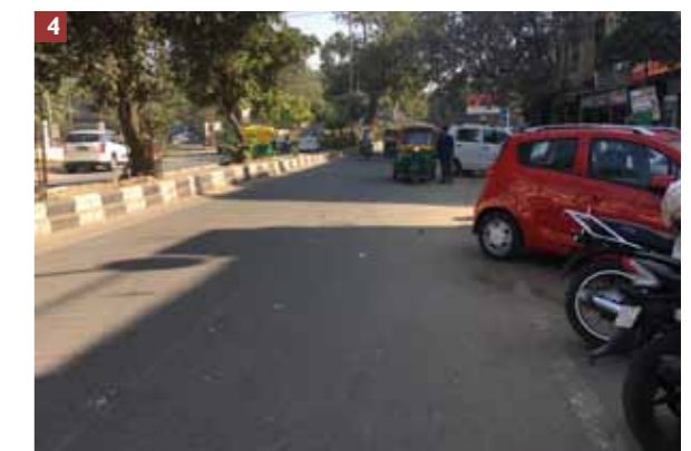
Street view showing under utilised road carriageway
