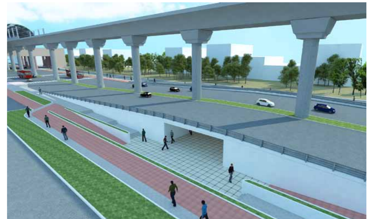
Aerial view showing the Grade separated Pedestrian crossing
