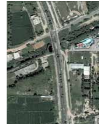
2006 - GT Road At Grade with unmetalled slip road for plot access
