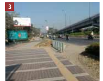
Broken bollards provide access points
