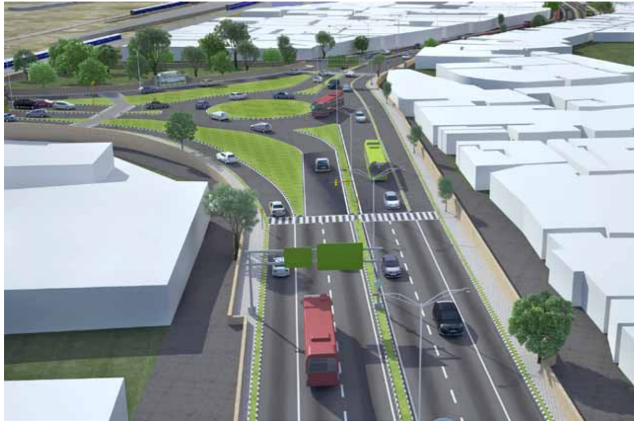
View of Kamal T-Point from Anand Parbat towards Sarai Rohilla Railway station View shows segregated lane for straight and left turning traffic at the junction and provisions for the Pedestrian crossing
