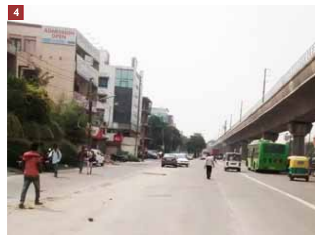
Absence of footpath
