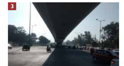
Image road section under the flyover
